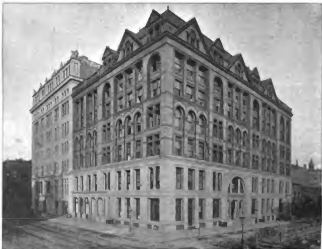
UNITED CHARITIES BUILDING, FOURTH AVENUE, NORTHEAST CORNER OF 22D STREET.
